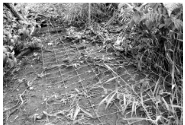
Fig. 3 The skirt of hogwire mesh added to a fence of the same material.
